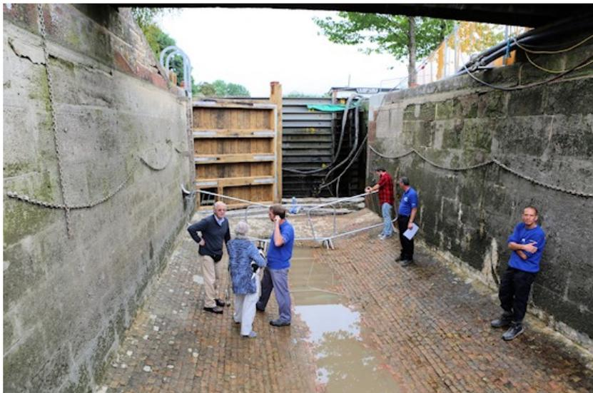
The original drawing of the lock showed that the pipe passed under the Sharpness Canal to a sluice in the wall just above a stop gate in the Whitminster pound of the Stroudwater Canal which is still in situ. This arrangement enabled the water level in the Whitminster pound to be lowered when needed for maintenance purposes.
