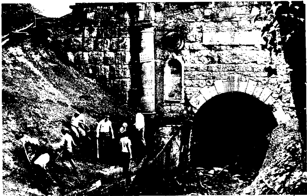
TOP PICTURE SHOWS THE CLEARED CANAL BED IN NOVEMBER. LOWER PICTURE IS OF FIRST WORKING PARTY STARTING IN SEPTEMBER.
