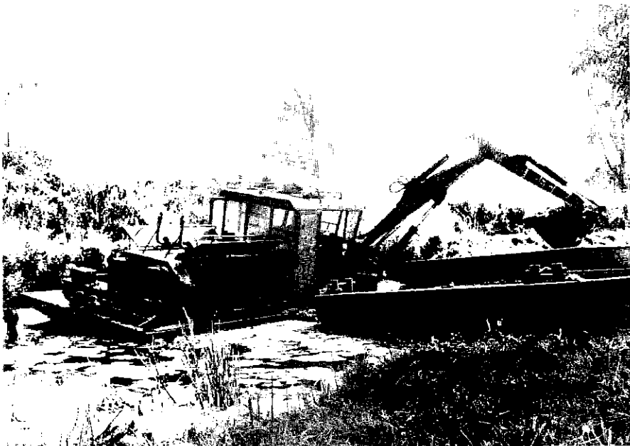
ACTION - HALF A TON OF SILT INTO THE BARGE
