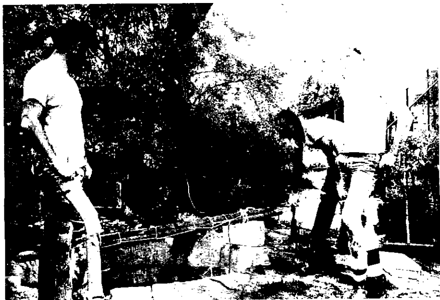
This is the newly discovered circular weir at Cerney Wick. The idlers are actually debating the best way of getting a large lump of concrete from twelve feet down, rather like one of those Krypton Factor larks.
