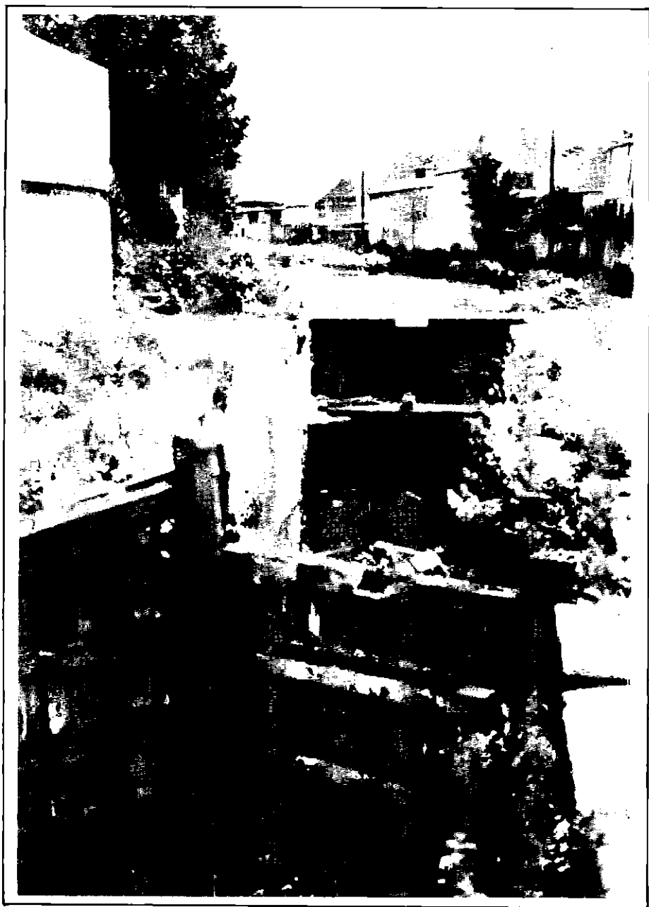
A sorry sight! The recent bypass work further up this pound has left this stretch of canal stagnant and the trip boat departure point deserted. Quite a contrast to the picture overleaf from two years ago
