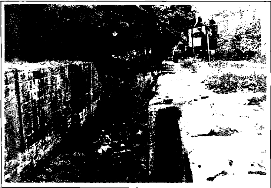
ABOVE: Volunteers eat away at the silt in the depths of Blunder Lock BELOW: The trusty Jones yard crane lifts another bucket of silt
