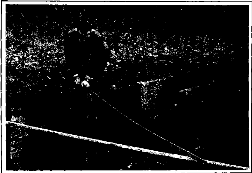
ABOVE: Cutting back the top gate mitre ready for timber facing BELOW: Rochdale Canal Workshops measuring up for bottom gates
