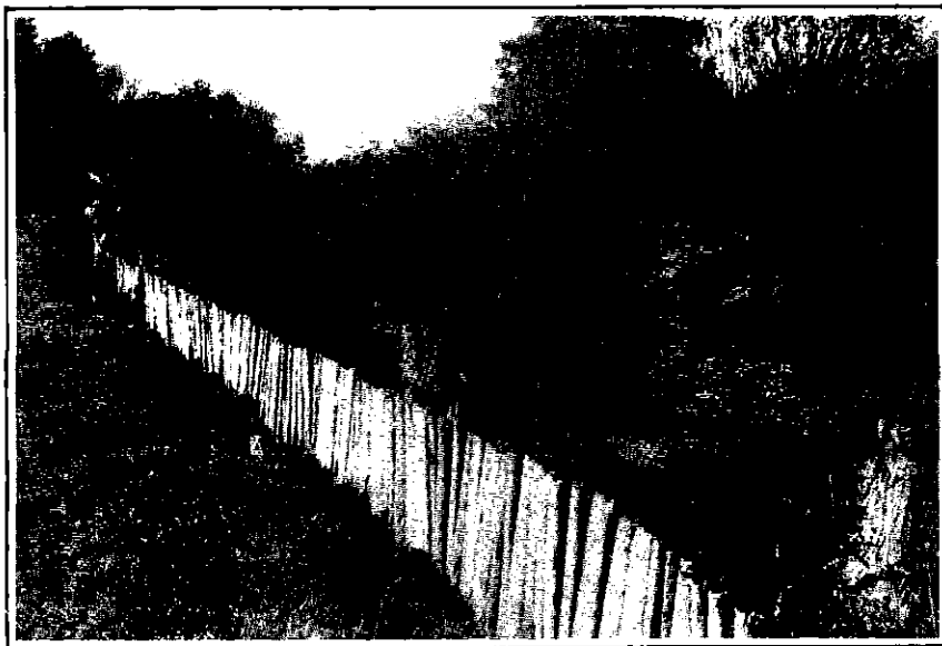
ABOVE: Timber stakes in place below Dock Lock ready to accept the infill BELOW: There goes the workshop - on its way to a new home at Toddington
