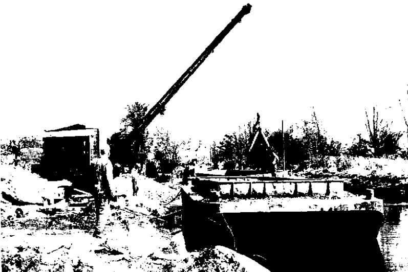
NEW DRAG LINE EMPTYING BARGE
