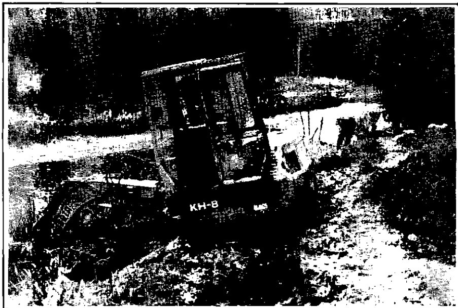
Tony Jones examines the breach at Wallbridge (Opposite) and gets stuck in (above) whilst the mini-digger lies idle!
