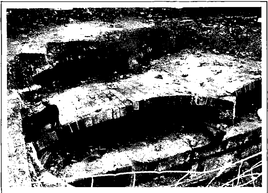
The Spill weir above Pike Lock.
